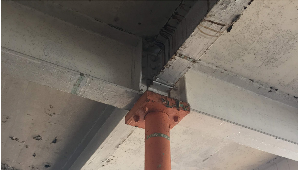
Existing steel column and slab support
