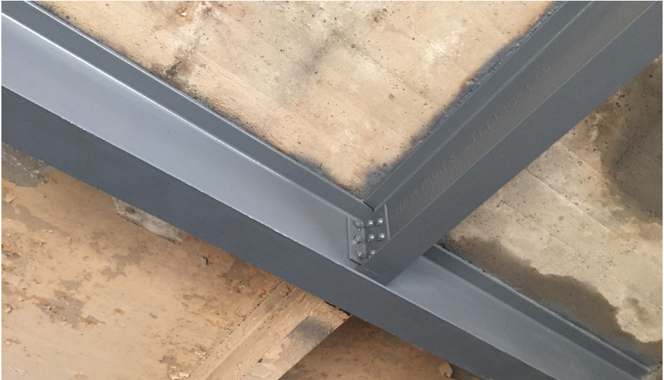
Sample of existing steel sand blasted and primed
