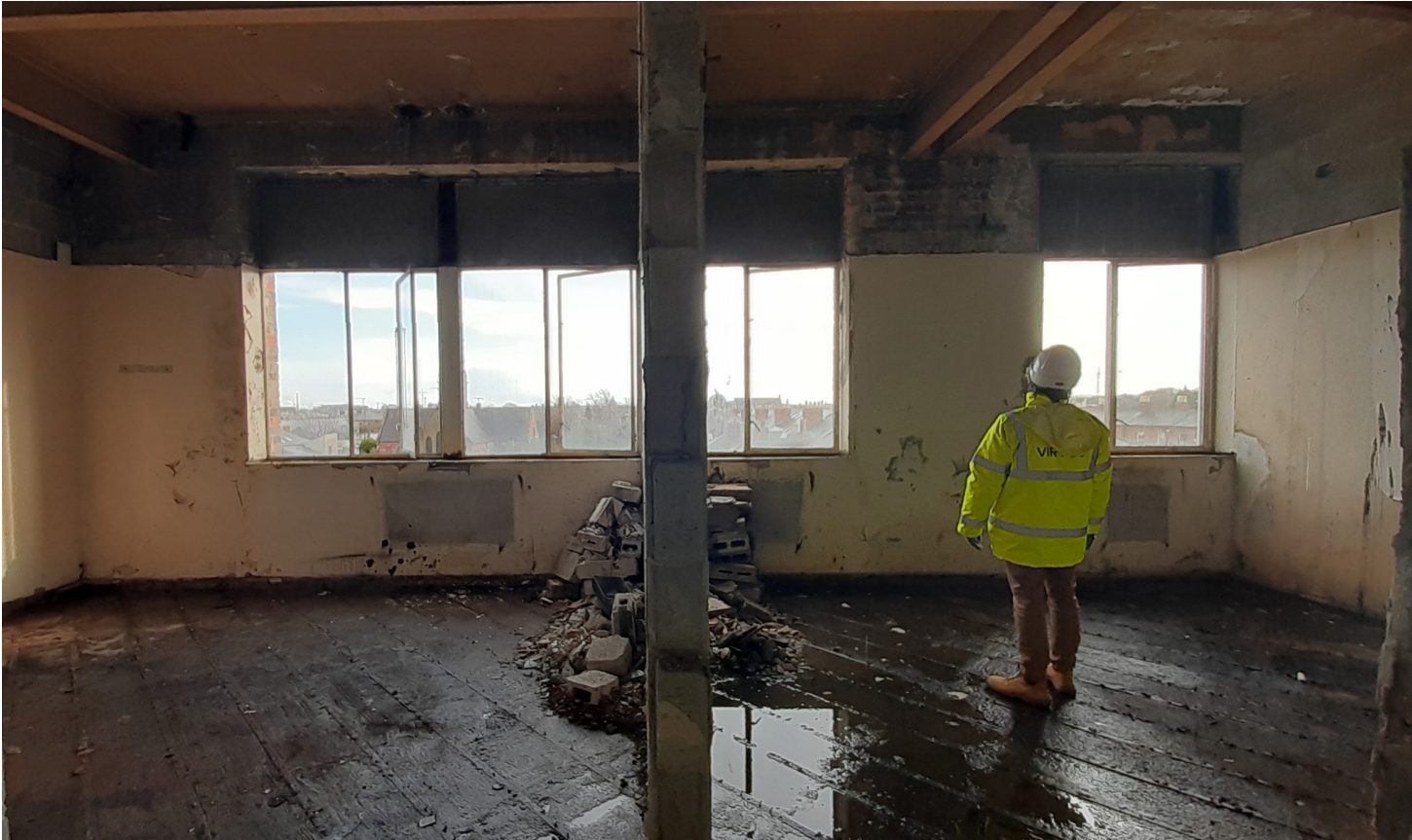
Existing Partition to Facade Interface
