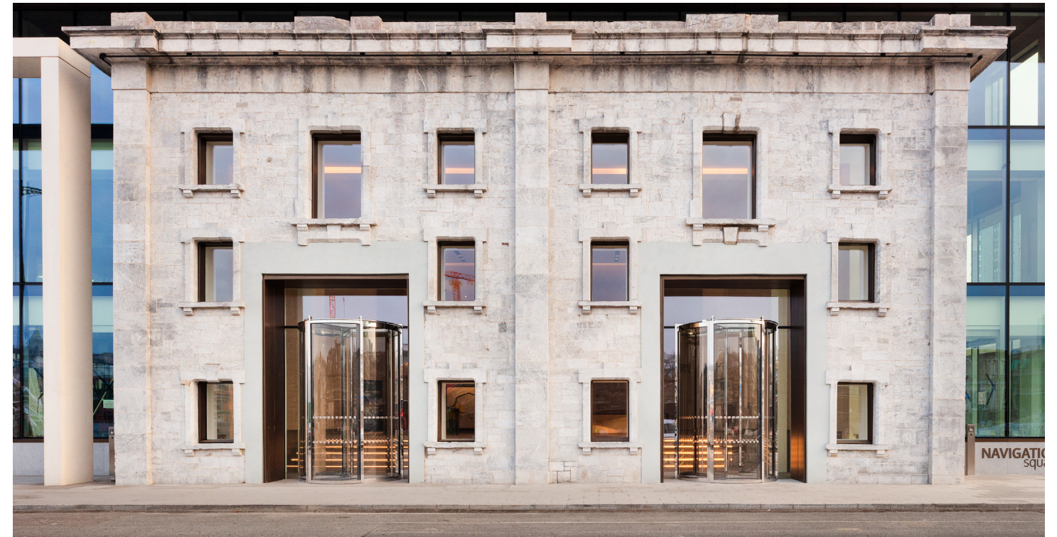
Albert Quay, Cork -HJLyons Architects - window surround to existing opes
